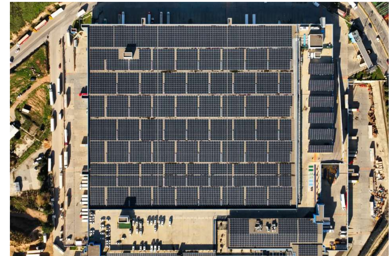
Lotus SPP - 40.000 m 2 Europe's Largest Green Facility with Storage Capacity
